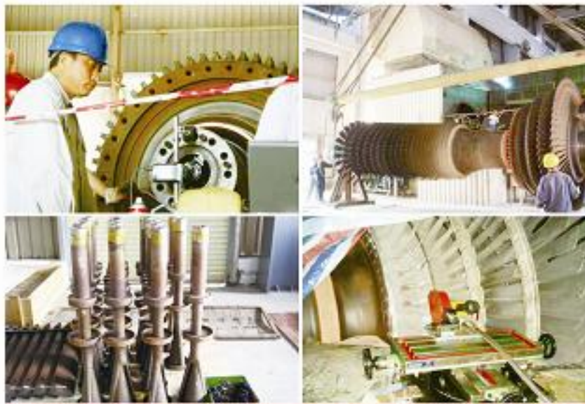
南光电力为深圳南光大港A88机组GT13E2型#5燃机 Overhaul by Nanguang Power of ABB GT13E2 #5 gas turbine unit for Shenzhen Nantian
