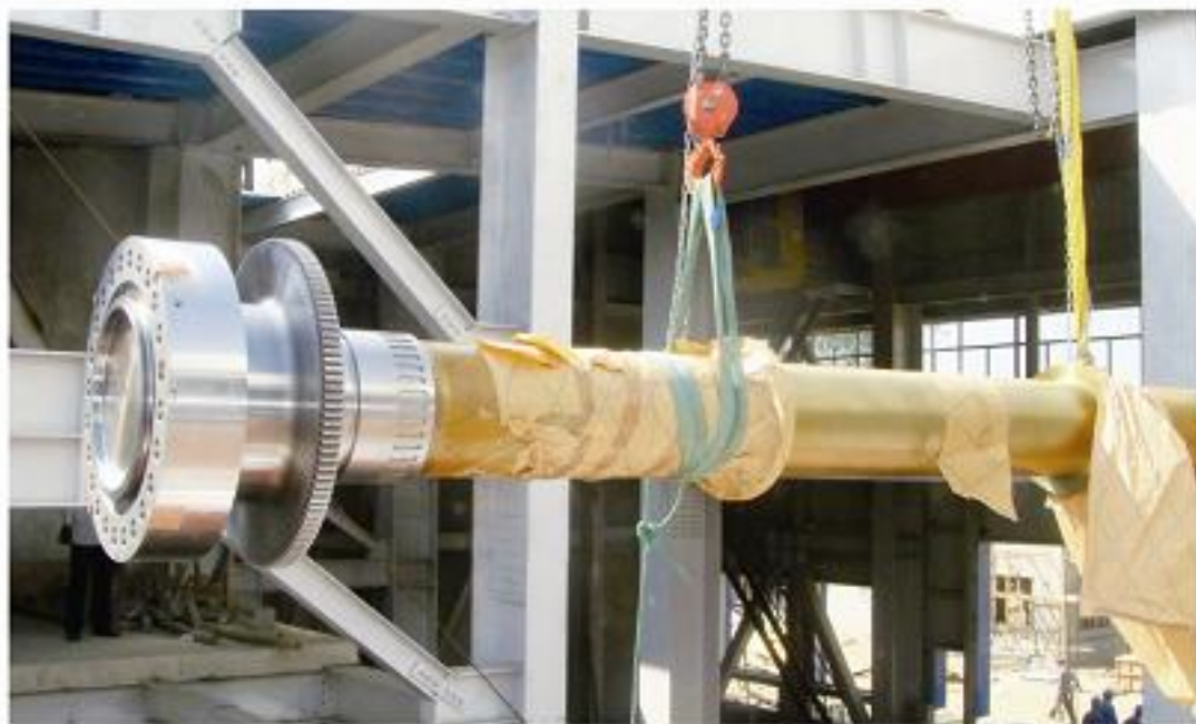
南博动力承接的孟加拉国大洛石卡巴哈燃气电厂V94.2燃机安装项目 Installation of Siemens V94.2 for SHIKALBAHA Gas Turbine PowerPlant in Chittagong, Bangladesh
