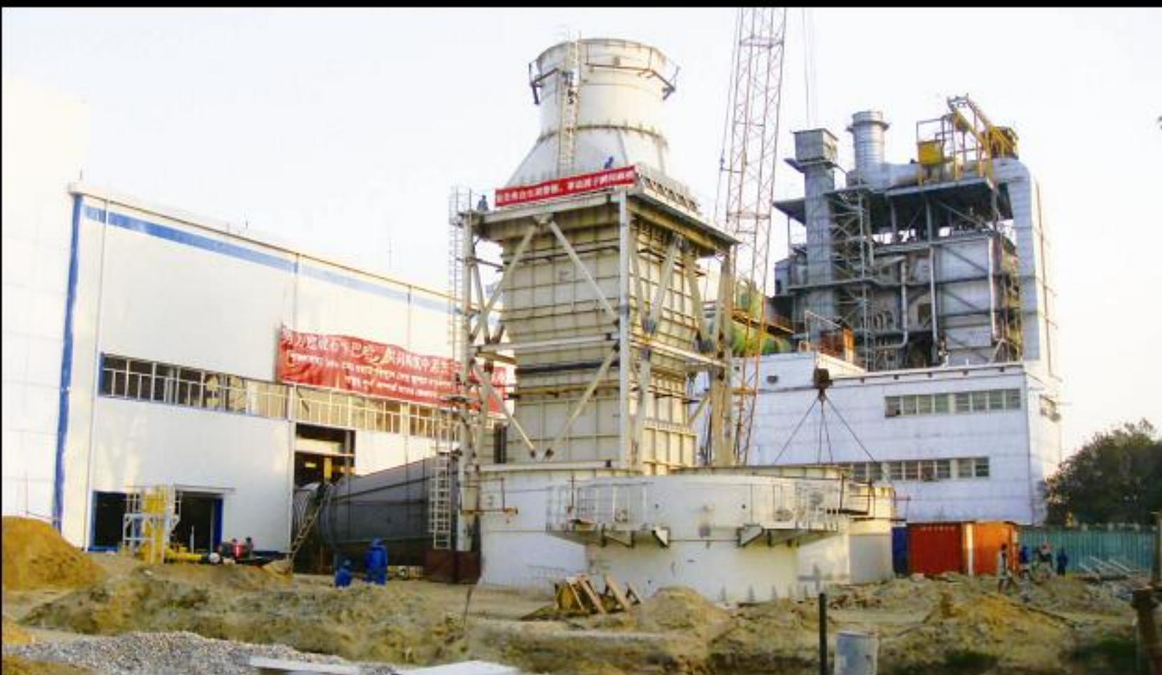
南瑞动力承建的孟加拉国南大港石卡巴堆燃气电厂西门子V94.2燃机安装项目 Installation of Siemens V94.2 for SHIKALBAHA Gas Turbine Power Plant in Chittagong, Bangladesh
